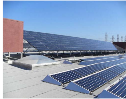
McCalmont Engineering designed this roof-mounted commercial solar system in Mountain View, CA, that produces 220 kWp for the Actel Corporation.
